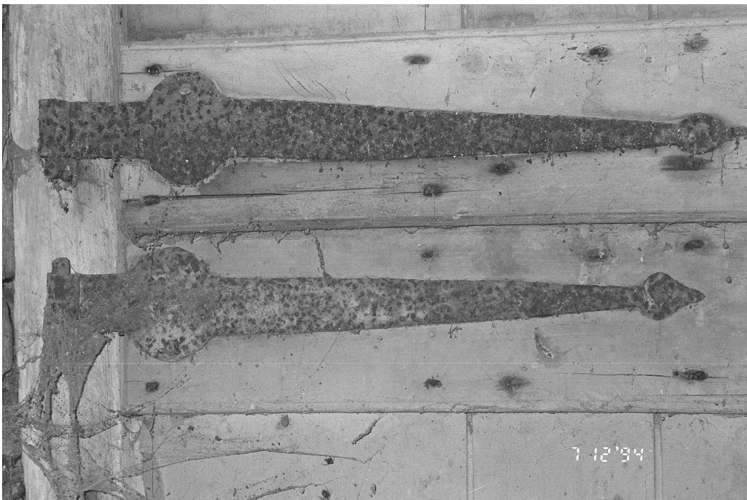
Photo 34. Detail of wrought iron strap hinges on interior of “Dutch” basement door at the McCutcheon House.
